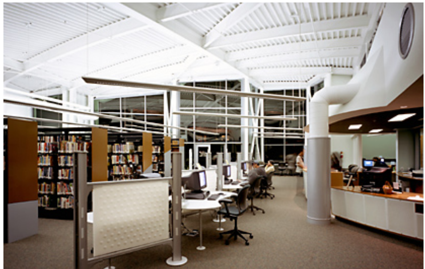
In the Cardiff-by-the-Sea branch library, the large duct at right provides supply air near floor level. Warm air is exhausted via the diffuser on the wall above the circulation desk. Photo by Frank Domin. Courtesy of Manuel Oncina Architects, Inc.
