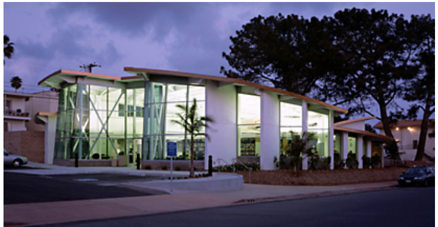
The Cardiff-by-the-Sea Branch of the San Diego County Library is one of a handful of new buildings in California with a displacement ventilation system.
